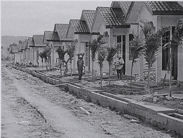
A NEW START IN INDONESIA — Recently built houses in Kajibu village in Aceh Province, the region that was hit hardest by the tsunami. Corruption and bureaucracy have been blamed for slowing the recovery process.
